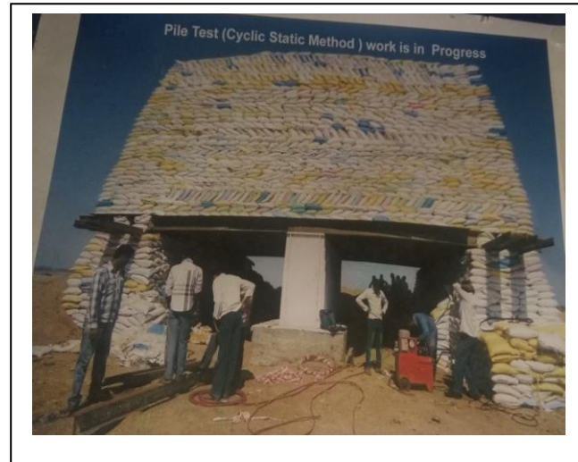
Fig 6 Details of pile testing
